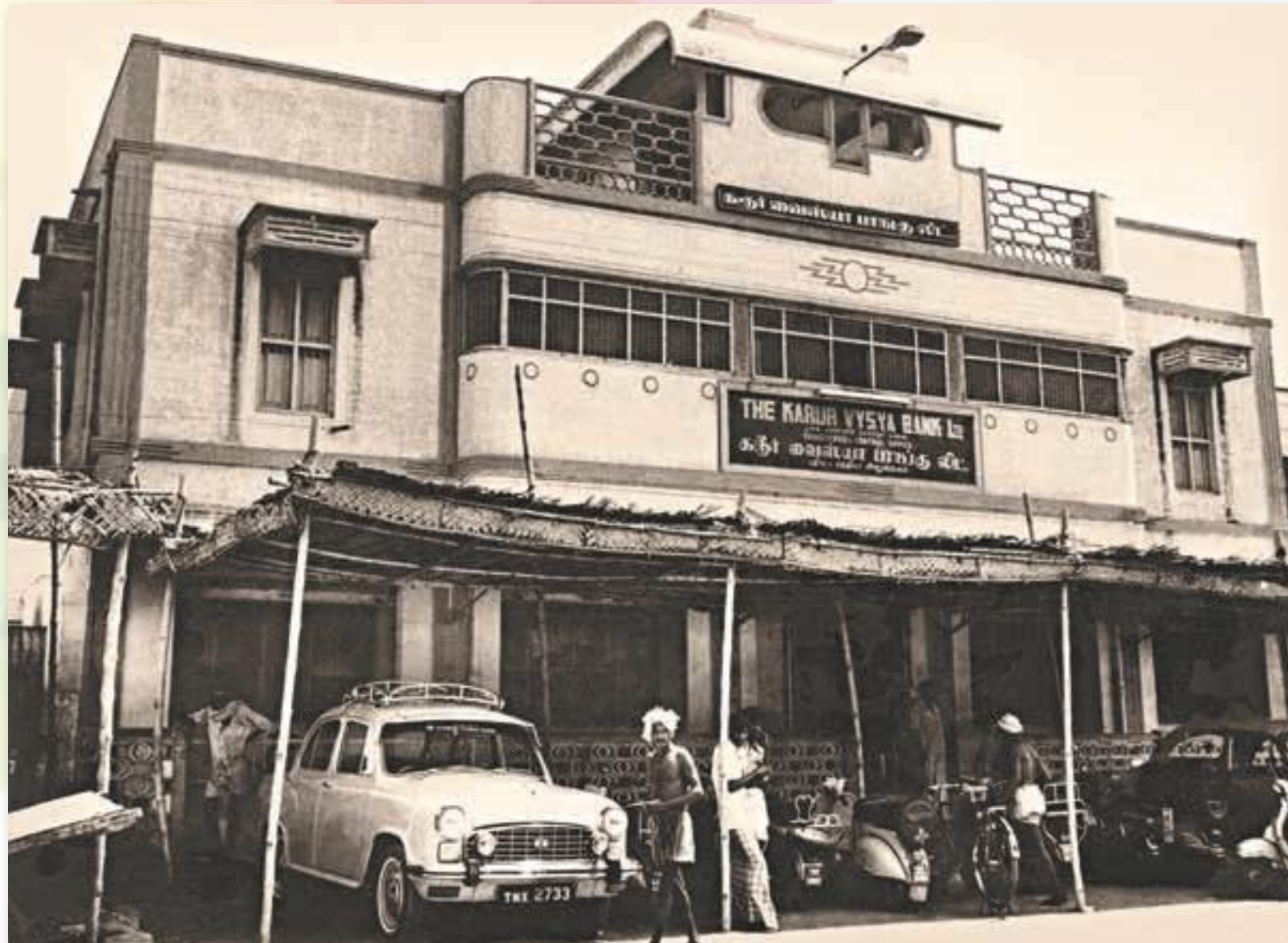
The Central Office at its old building, Karur
