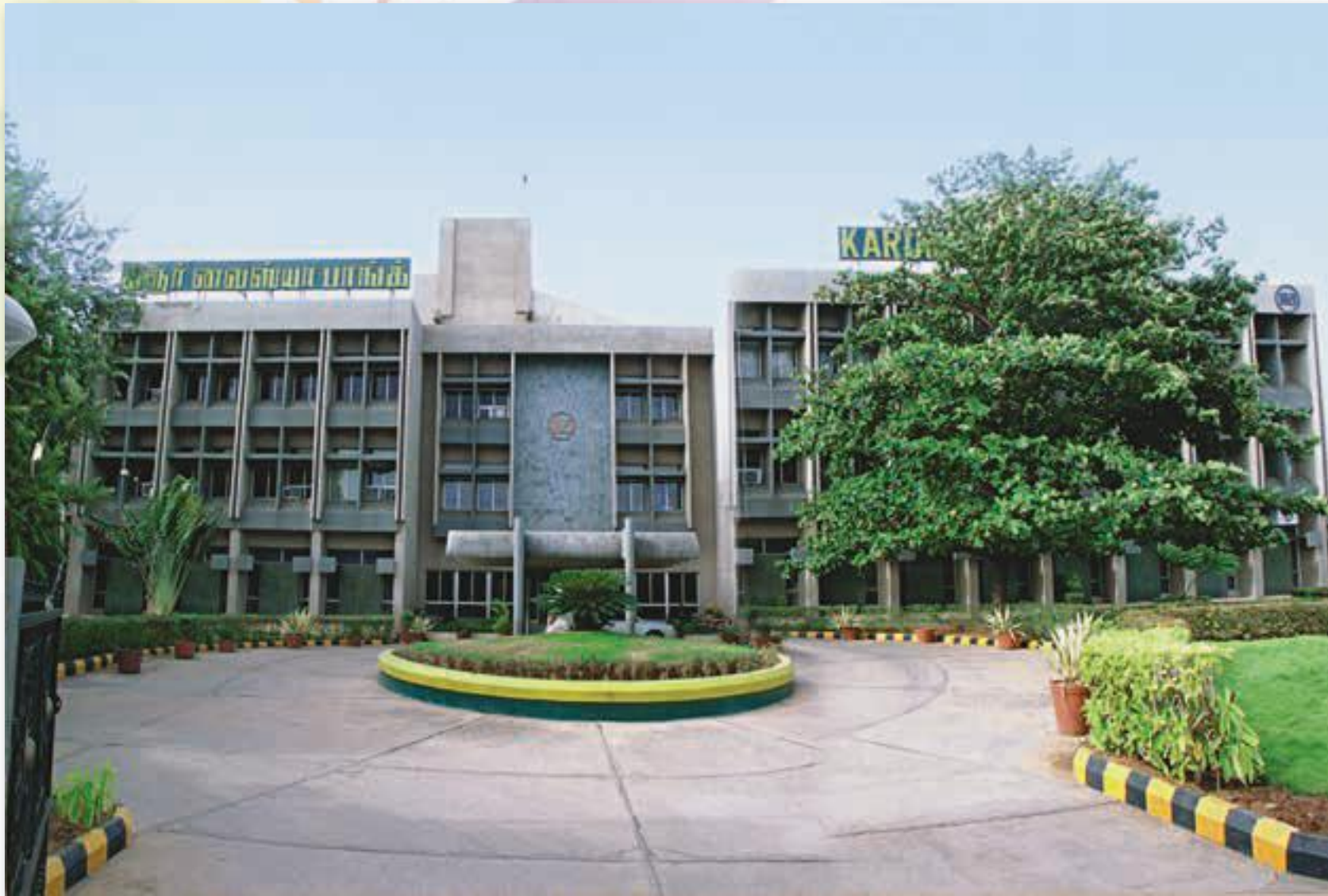
The new Central Office, Karur, inaugurated in 1983
