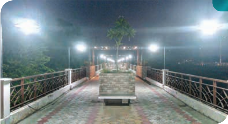
Old Amaravati Bridge after the makeover
